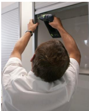
Image 7: Remonter le rail de guidage
